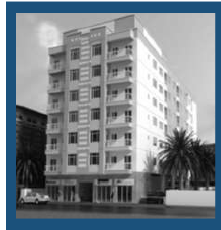
PROJECT: Residential & Commercial Building BF+GF+6Typ Fl+GymFl+Roof Area: AL BARSHAA – Plot: 3734258 DUBAI – UNITED ARAB EMIRATES CLIENT: Mr. Sultan AHMED ALALY
