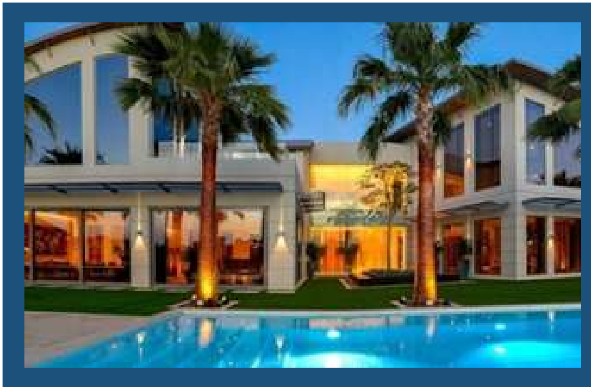
Project: PALM JUMEIRAH - RESIDENTIAL VILLA-Plot no. (PJJPJ J09)- PALM JUMEIRAH-DUBAI CLIENT: POINTE INVESTMENTS LIMITED CONSULTANT: CROWN ENGINEERING CONSULTANT ENG.
